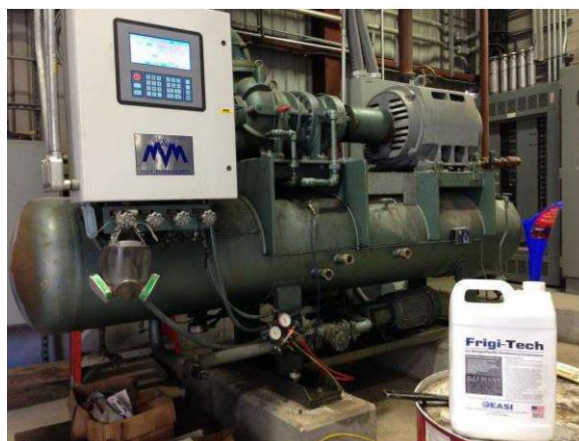
Frigi-Tech will cause the insulating layer of oil to return to the compressor sump and no longer build up on heat transfer surfaces
