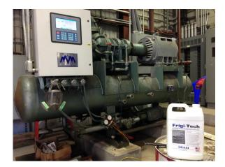
Frigi-Tech will cause the insulating layer of oil to return to the compressor sump and no longer build up on heat transfer surfaces
