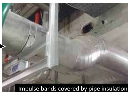
Impulse bands covered by pipe insulation
