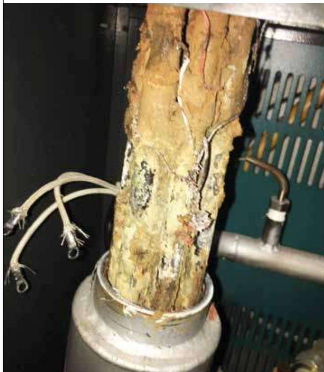
Untreated heat exchanger for 3 years.
