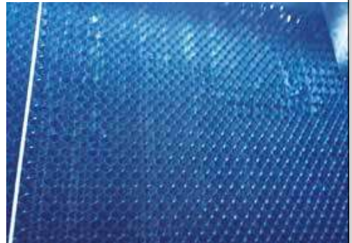
The inside of CT-1, after 3 weeks with Vulcan. It illustrates clean flutes that are in constant contact with Vulcan-treated water and a few dry (untreated) areas that still have some remaining green biofilm.
