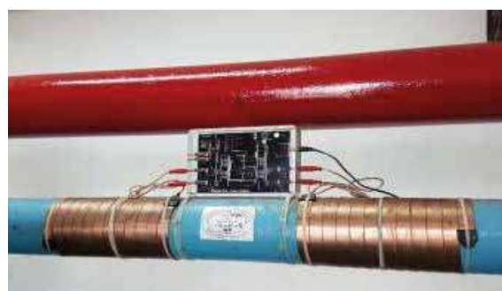
Anti-Scale System Vulcan S25 installed
