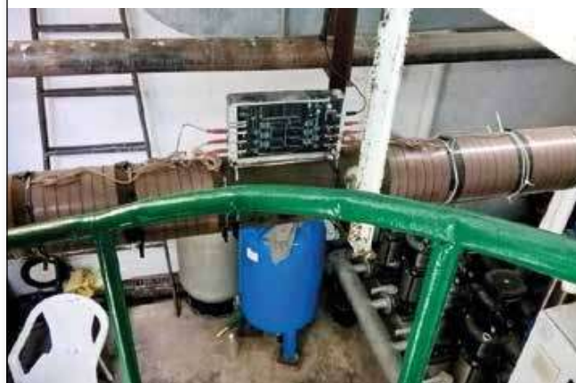
Two Vulcan S100 were installed.
