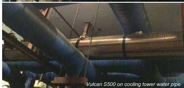
Vulcan S500 on cooling tower water pipe
