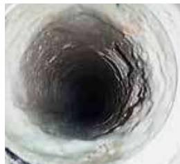
2 weeks after Vulcan was installed, scale had been softer and fallen out.
