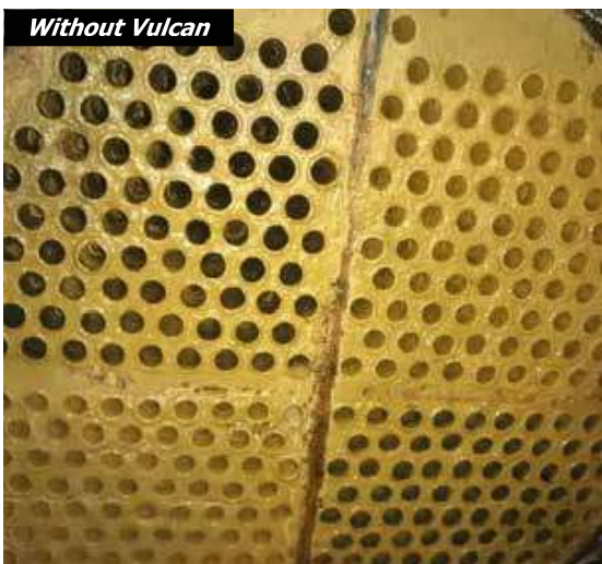
Before installing Vulcan, the scale was very thick and hard in the heat exchanger tubes.
