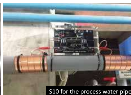
S10 for the process water pipe
