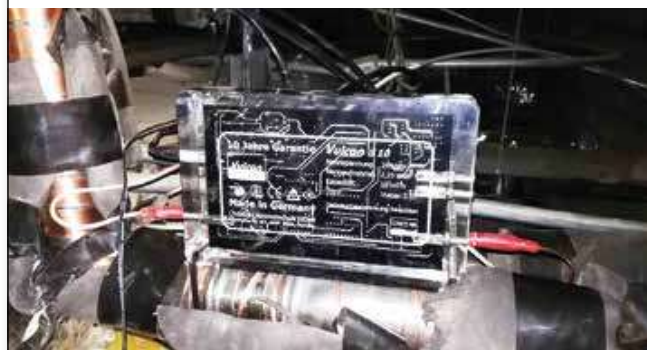
Vulcan S10 was installed on the main water line of the Chinese kitchen.
