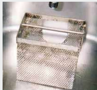
Grease trap was cleaned with water flow under the sink.
